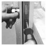
Screw sleeve nuts to the door with two M5 x 45 screws. Apply a light pressure to the support plates.
